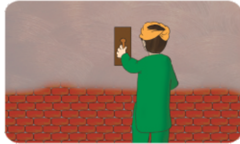
A mason plastering with a 'garmala'.
